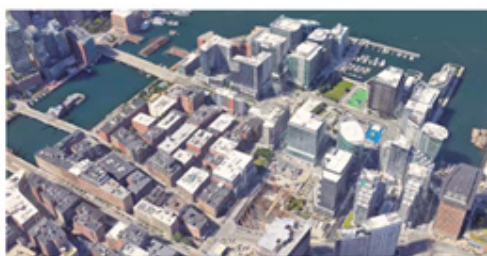
Fig. 1. The Development of Boston Seaport Innovation District between 2010 and 2020. Source: Google Maps.
